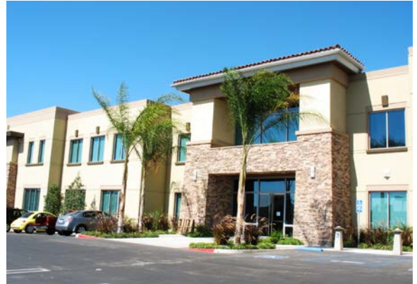
Office complex in Rancho San Diego
