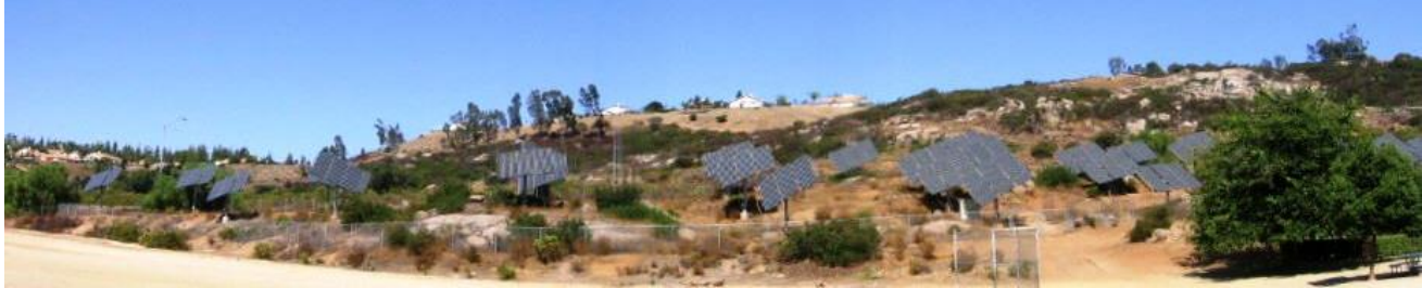
Solar panels in Alpine
