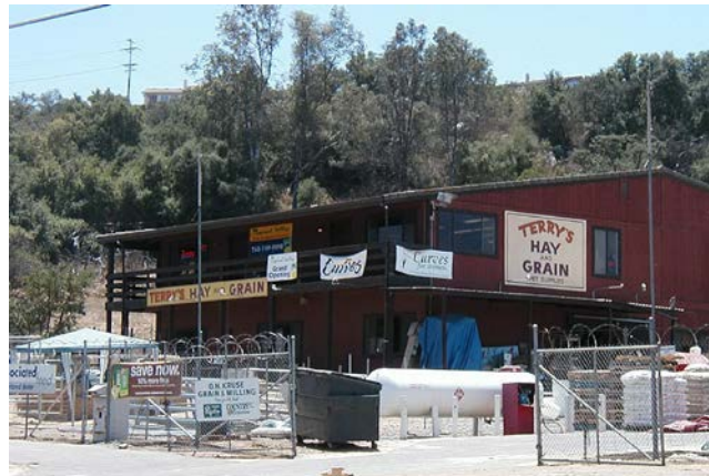
Rural Commercial use in Valley Center
