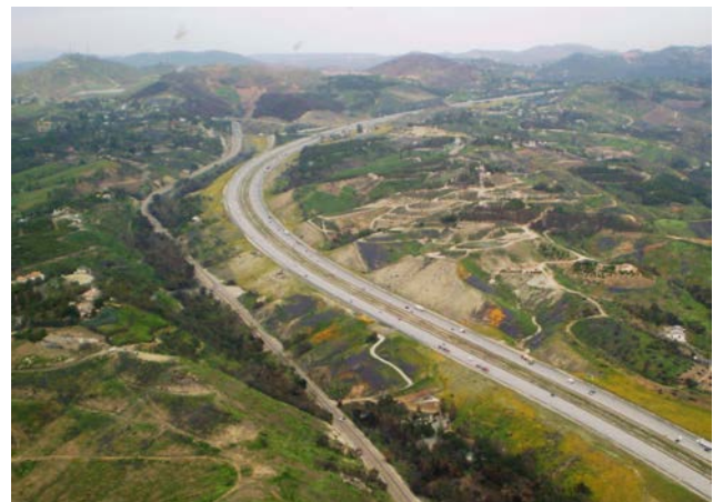
Interstate 15 looking north
