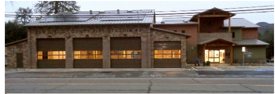
Fire Station in Pine Valley
