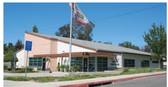
Fallbrook Sheriff substation
