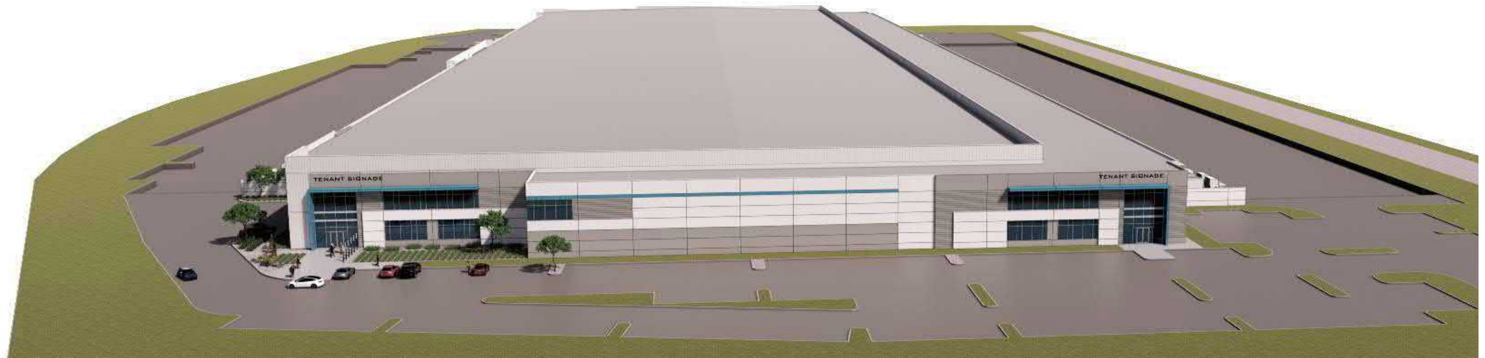
Aerial View of West Elevation
