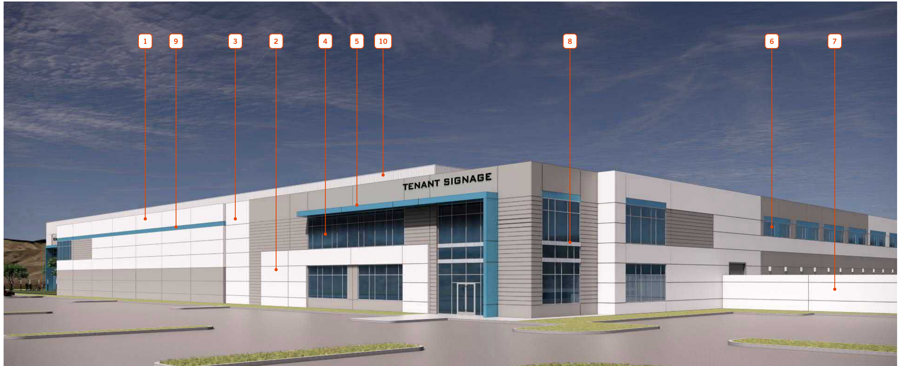
View at South West Office Component
