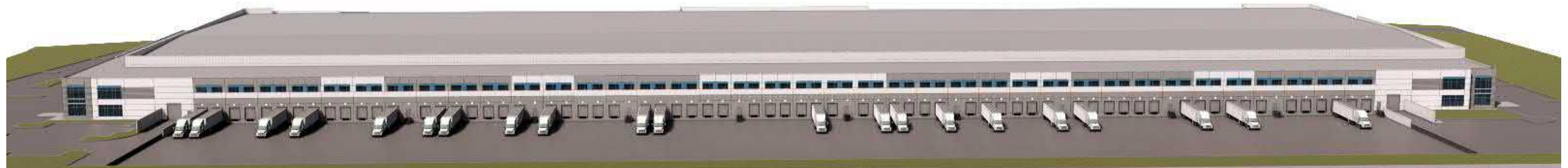
Aerial View of South Dock Facing Runway
