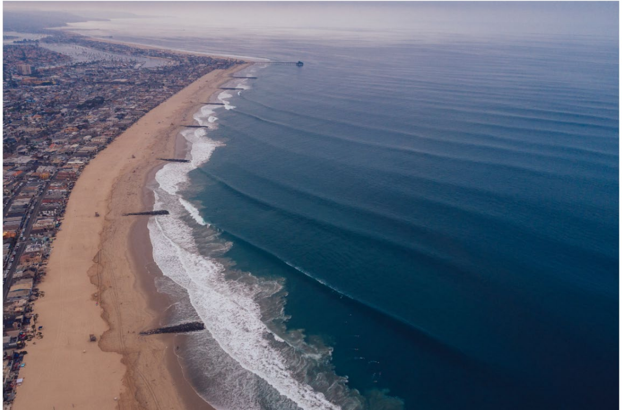
Figure 2-13. West Newport Beach Groins - South (DBW & SCC, 2002)
