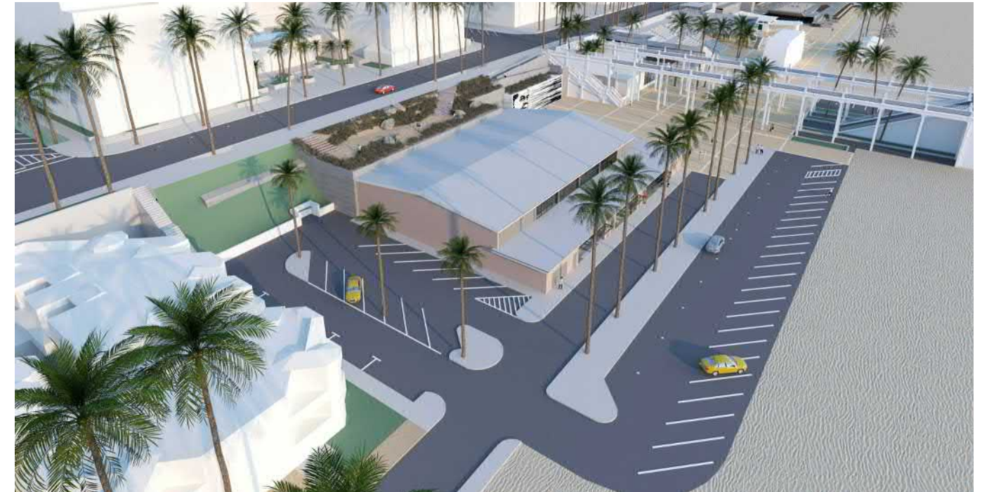
OPTION B RENOVATION/MODEST ADDITION This view illustrates a modest single story addition on the east side of the building, which includes a rooftop park on top of the addition. Also included is a more extensive interior renovation to enlarge classrooms, which would require structural upgrade.
