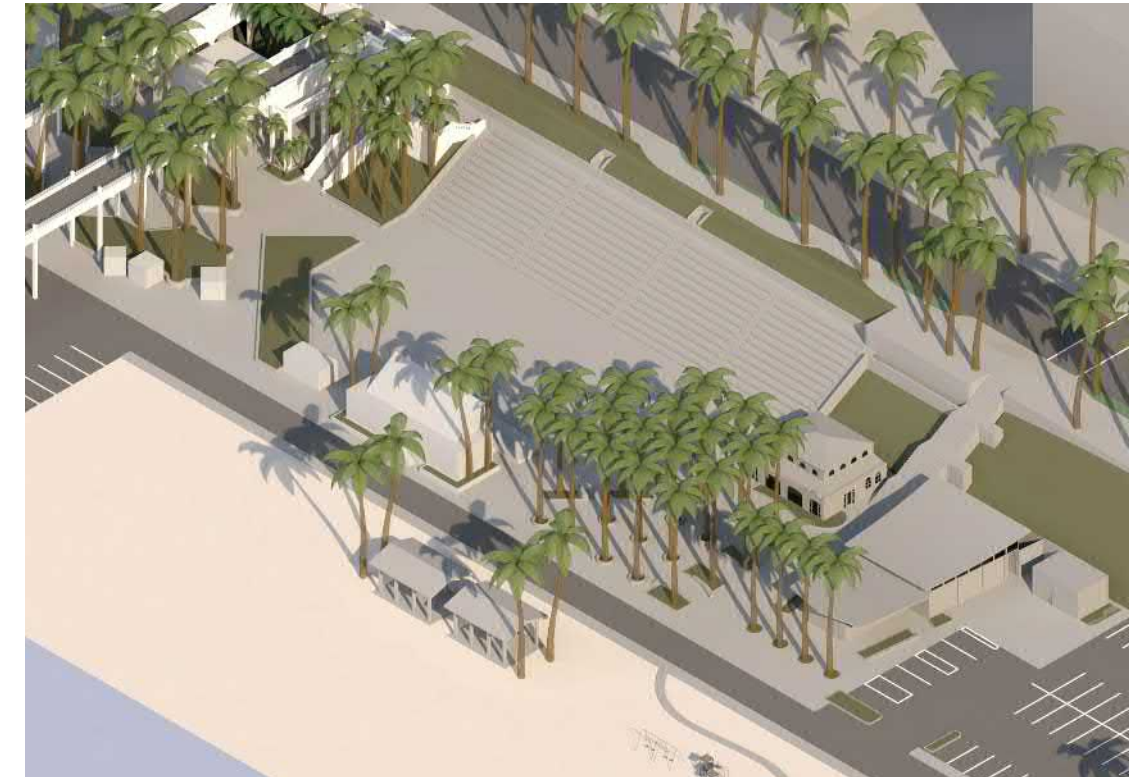
JUNIOR SEAU PIER AMPHITHEATER AND BANDSHELL The amphitheater venue seats approximately 2,500 people. 1,500 are seated in the stepped concrete seating area. Approximately 1,000 can be accommodated in the open area between the amphitheater seating and the bandshell.
