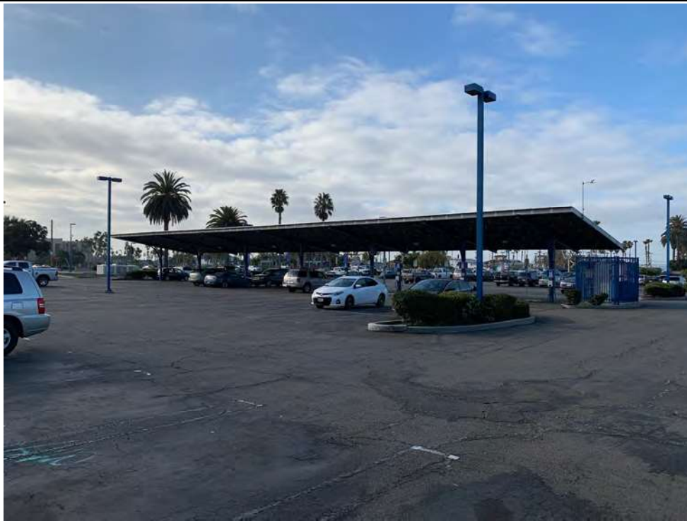
Photo #1 View of the solar charging station located in the east central portion of the Property.
