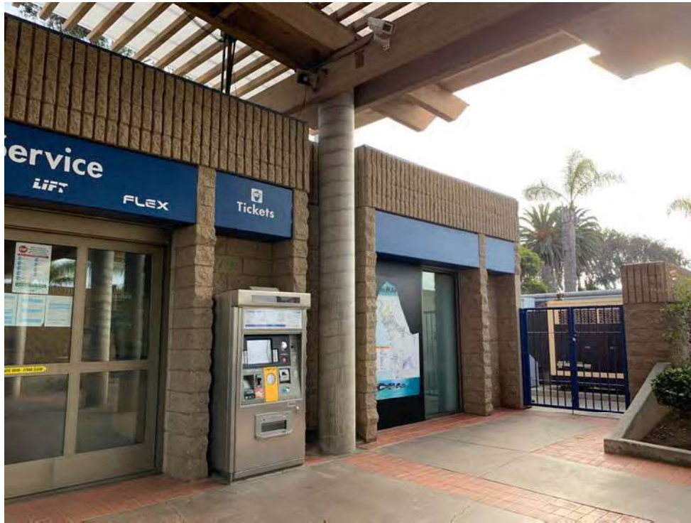
Photo #3 View of the customer service building in the eastern portion of the main building and an exterior locked enclosure with a generator and electrical switches.
