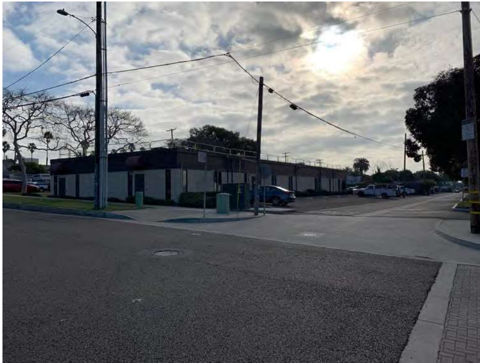
Photo #5 View of the North County Transit District office building and transformer located in the southeastern portion of the Property.
