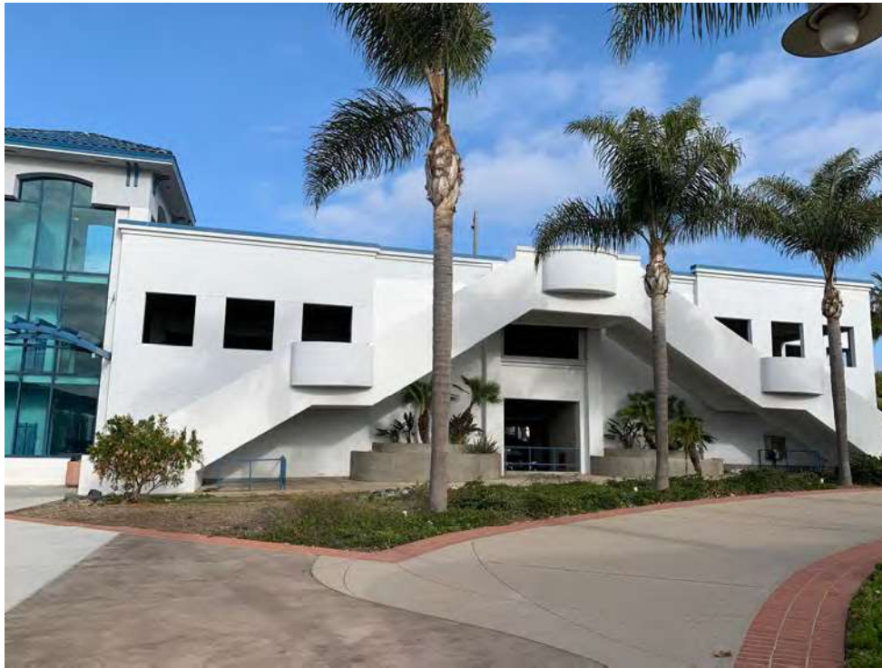
Photo #9 View of the adjacent parking structure to the northwest.
