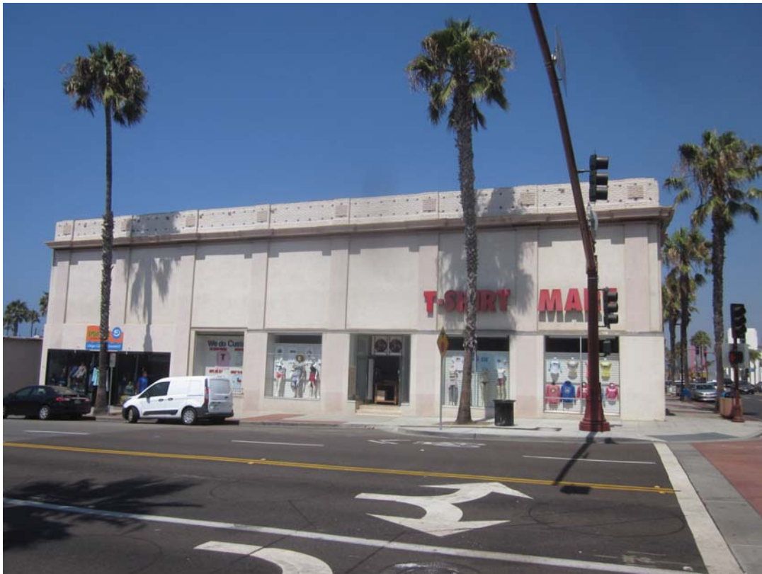
Overview of 201 Coast Highway (view to north)
