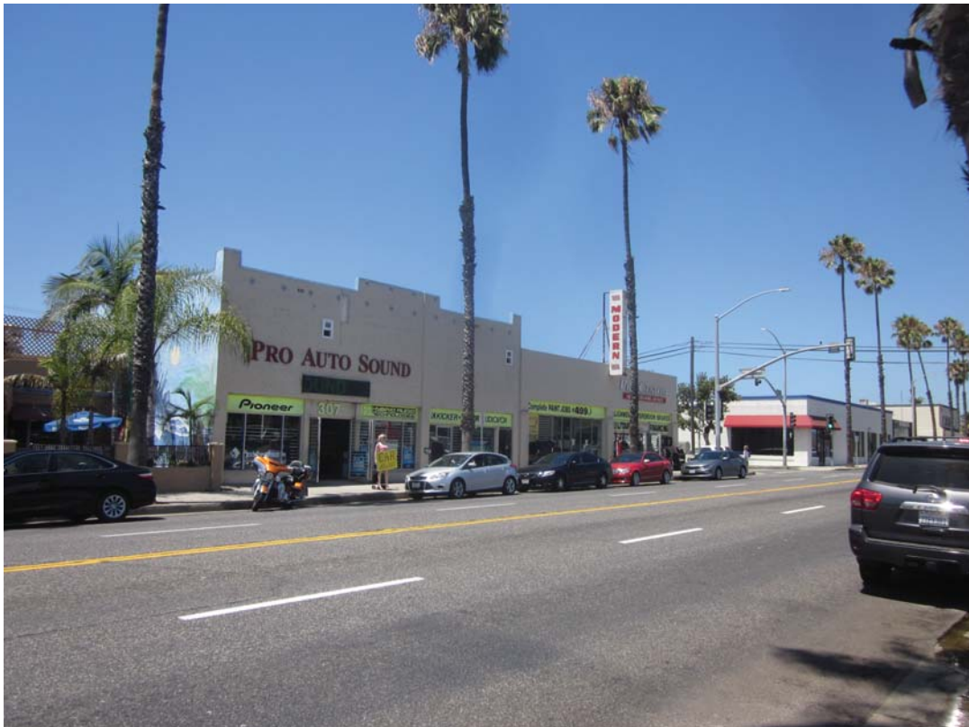
Overview of 301 Coast Highway (view to NW)
