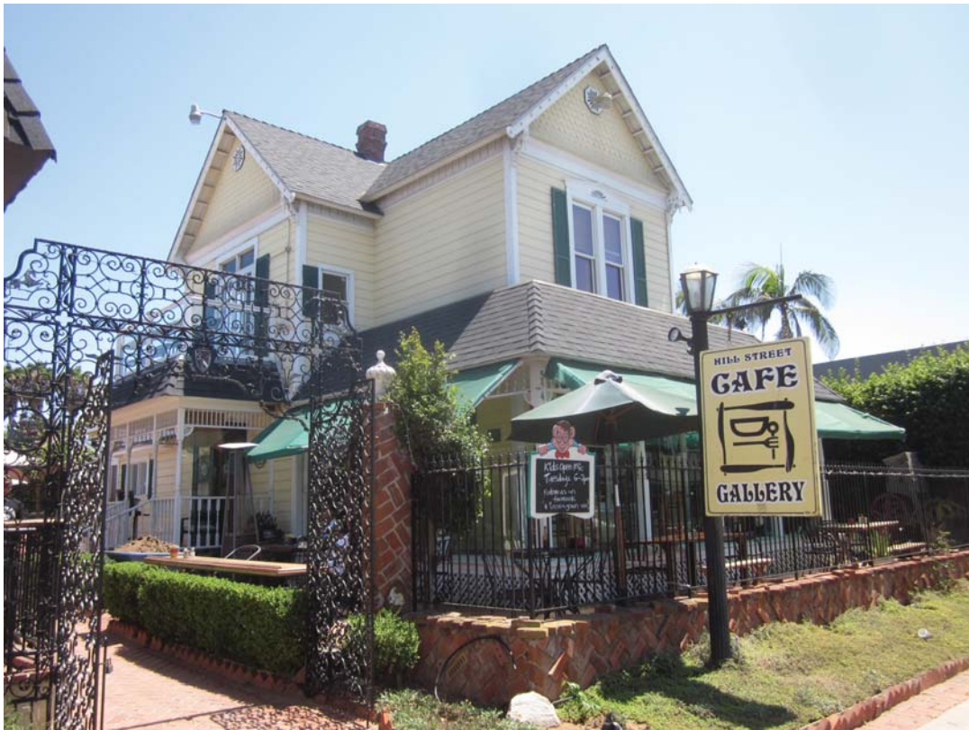
Overview of 524 Coast Highway (view to SE)
