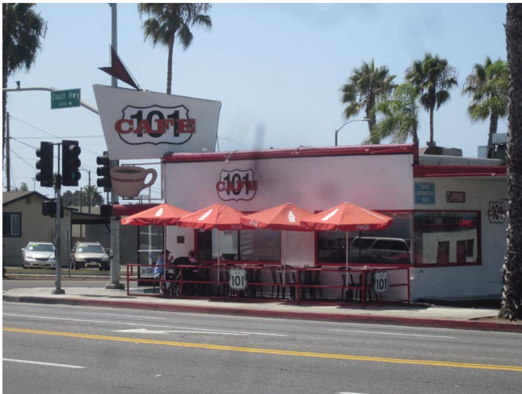
Overview of 631 Coast Highway (view to west)
