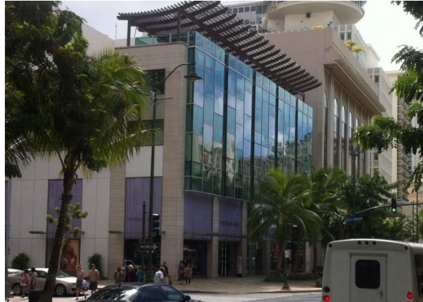
Example of Public Parking Structure
