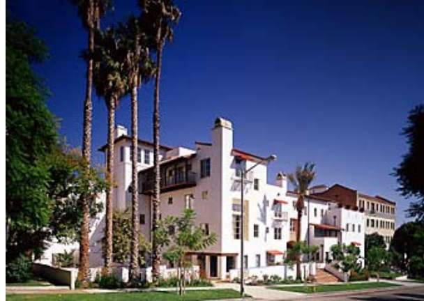
Example of Podium Building
