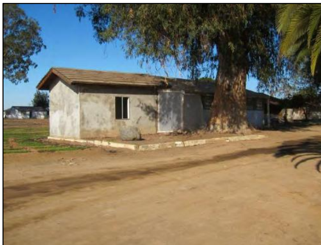
Building 5: storage (appears to be relatively recent)
