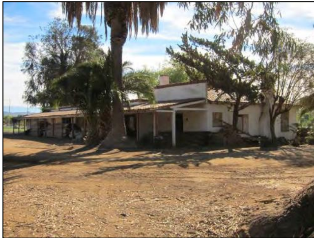
Building 4: residence (circa 1930s)
