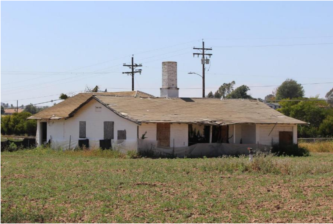
Figure 16 Residence, view looking northwest. (IMG_8709)
