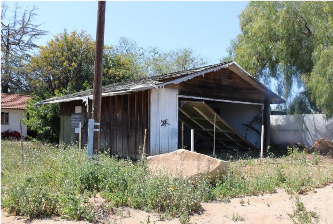
Figure 5 Garage building, view looking northwest. (IMG_8496)
