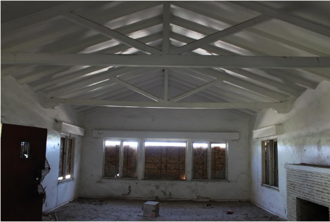
Figure 10 Interior of Great Room, western portion of the building, view looking south. Notice the Spanish Colonial Revival style influences in the iron grille door insert, chamfered king post trusses supported by ogee corbels, and exposed beams. (IMG_8588)
