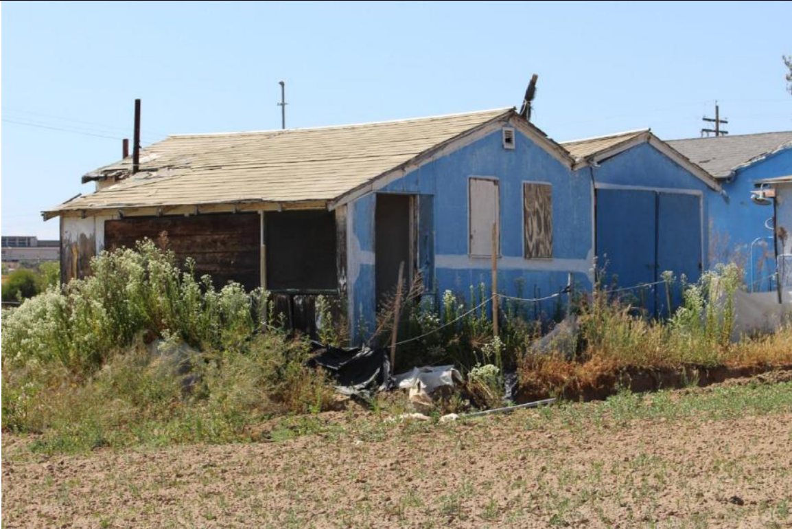
Figure 14 Residence, view looking northwest. (IMG_8695)
