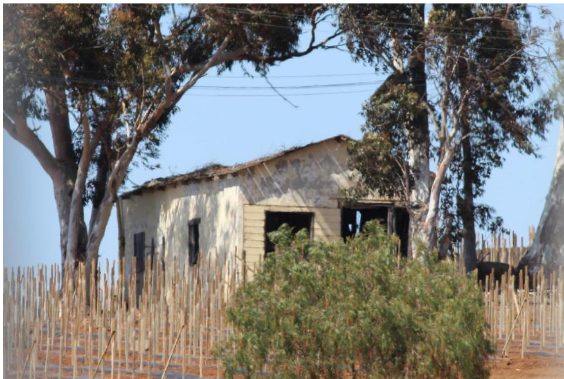
Figure 18 Residence, view looking north-northeast. (IMG_8746)
