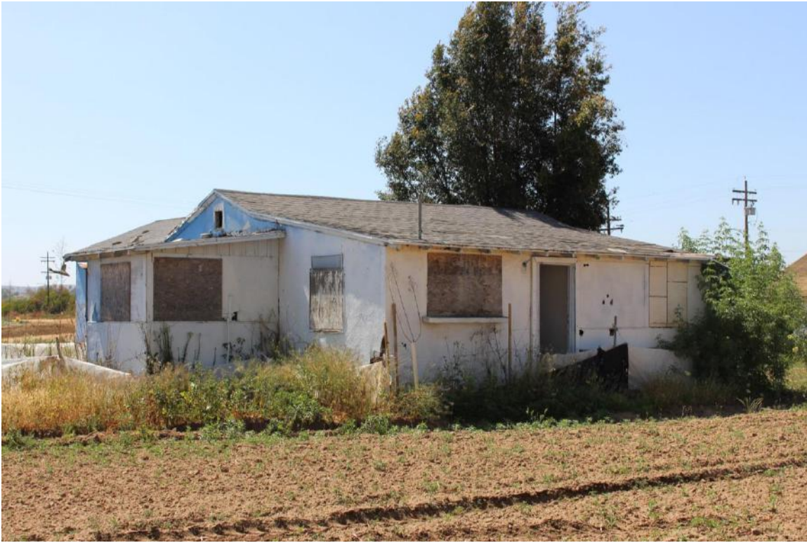
Figure 15 Residence, view looking northwest. (IMG_8702)
