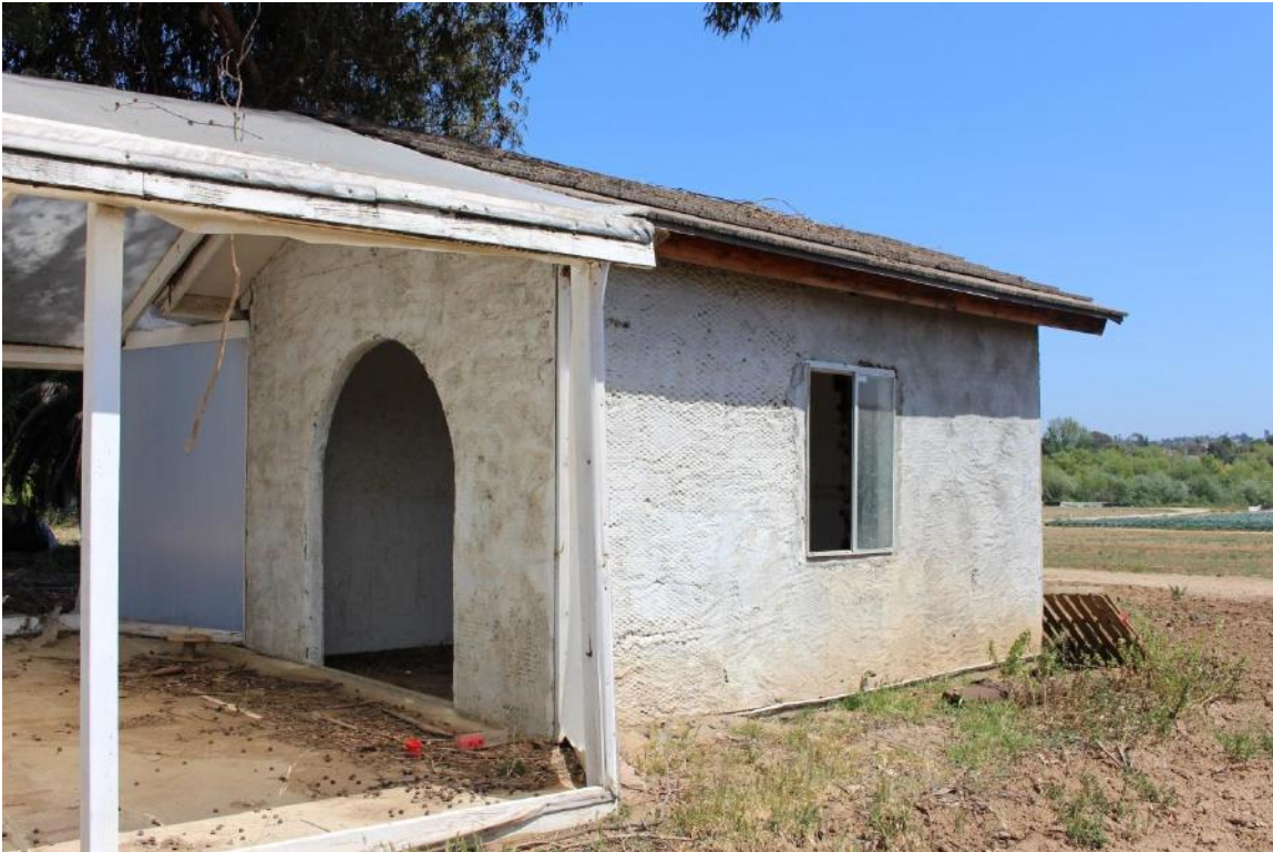
Figure 11 Small miscellaneous building, view looking southeast. (IMG_8646)
