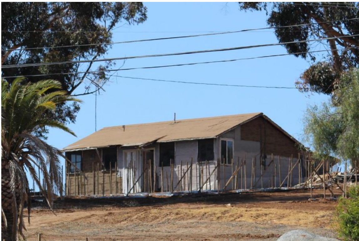
Figure 17 Residence, view looking northwest. (IMG_8740)
