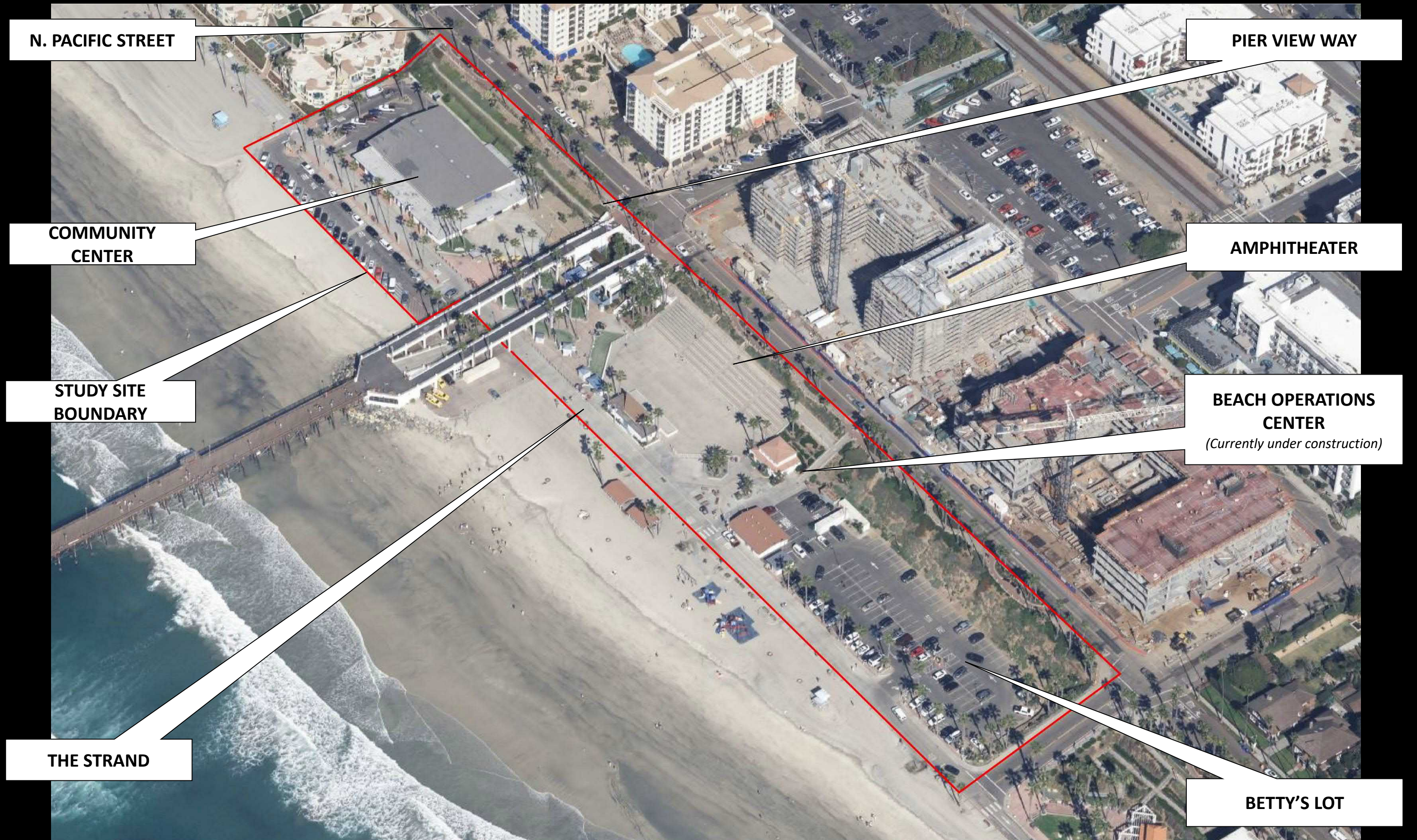
FEASIBILITY STUDY SITE– VIEW FROM SOUTHWEST
